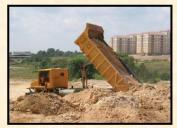
called cut volume. Importing suitable land and materials can be expensive because contractor needs to source the import materials. Suitable materials may at far away from project site and increase the transportation cost. Disposing extra material can be expensive by searching for suitable location for dumping.
